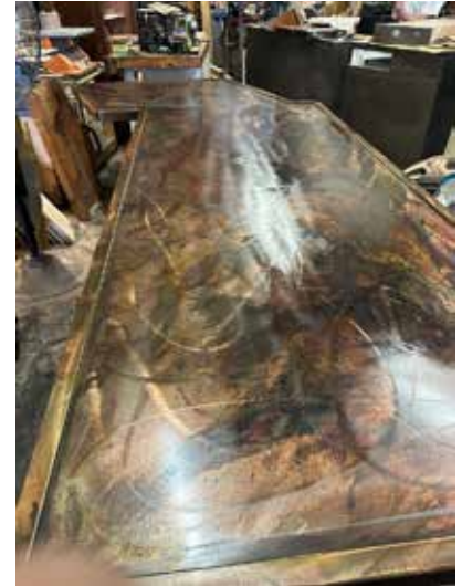
Bar top, 16 gauge steel with Steel FX pantina.
