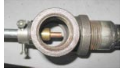
Figure 15: A “T” burner with tip 1” from junction
